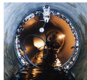
Sewer rehabilitation (image)
