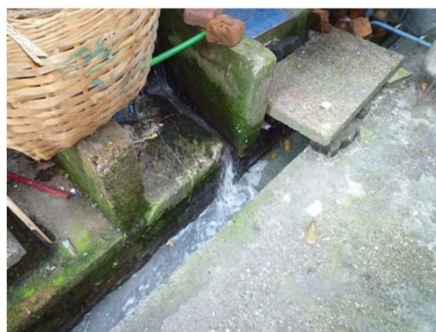
Discharge of domestic wastewater to stormwater canals in Yangon City
