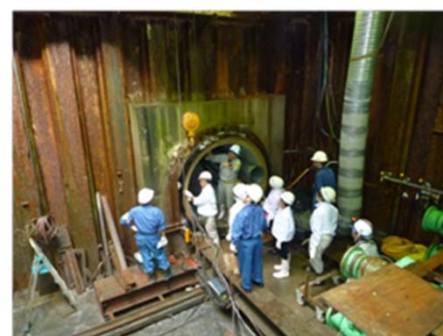
Pipe jacking construction site in Osaka City
