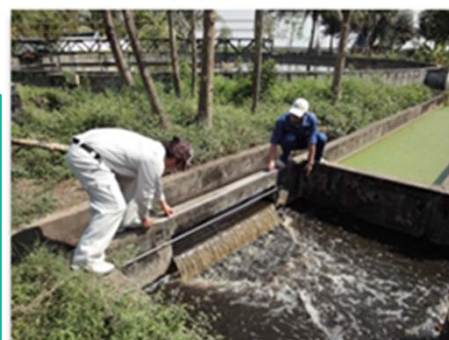
Site survey of a sewage treatment plant in Yangon City
