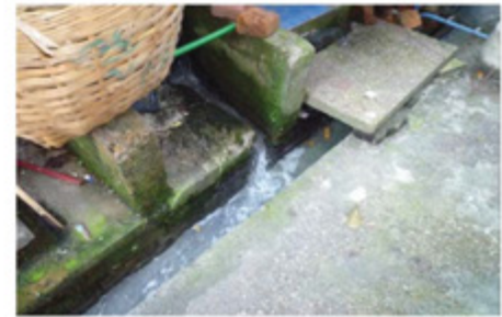
生活排水の雨水排水路への放流 Discharge of gray water into a side ditch
